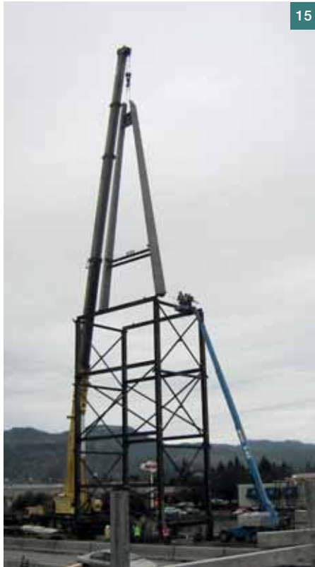
Fig. 16 I-5 Bridge, erection sequences: a) segment erection, b) closure, c) deck casting and prestressing
